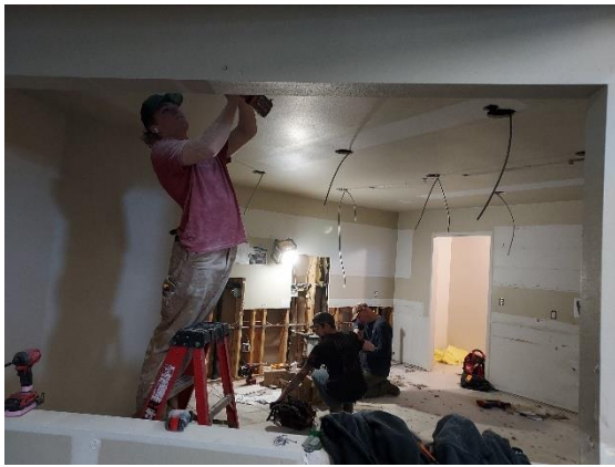
Apr 22-30 Electricians in first installing recessed lighting. Drywalling next then painting.
